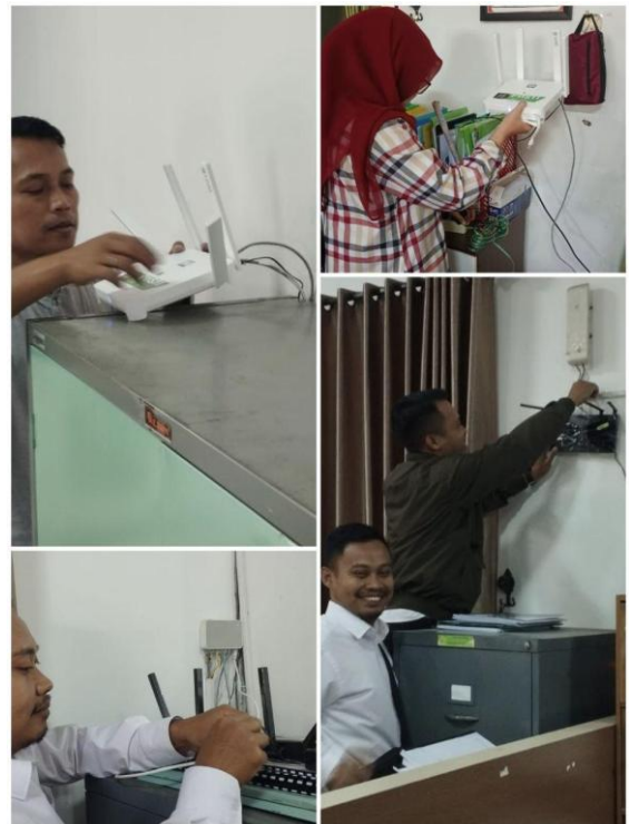
Gambar 16. Gambar Proses instalasi Access point / Router Wifi di Ruang Prodi
