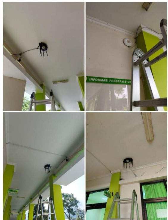
Gambar 17. Gambar Proses instalasi Access point / Router Wifi di Ruang Kelas
