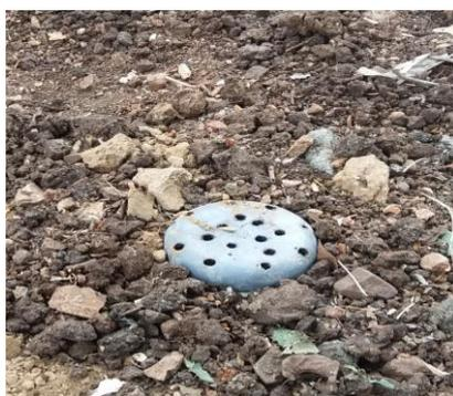
**Gambar 2.** Lubang Resapan Biopori
