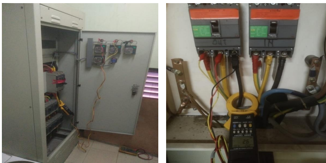
Figure 2. The process of measuring harmonic content with a harmonics analyzer
