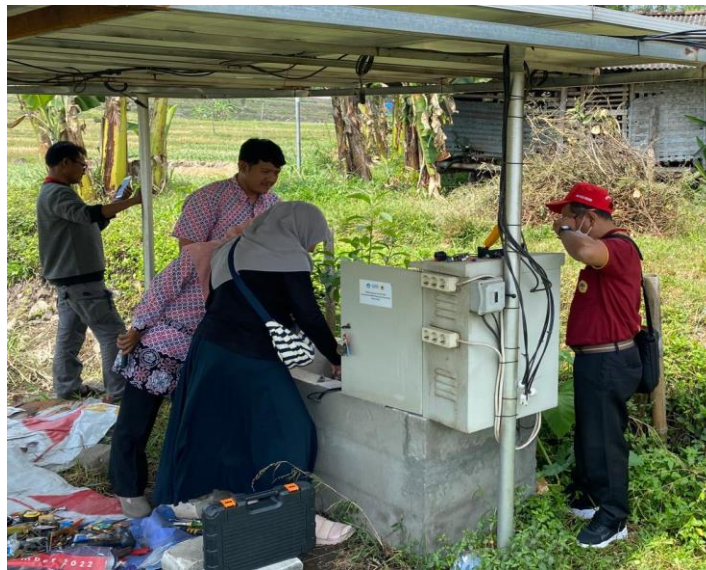
Figure 5. Cleaning Inverter Panels from Wild Ant Nests
