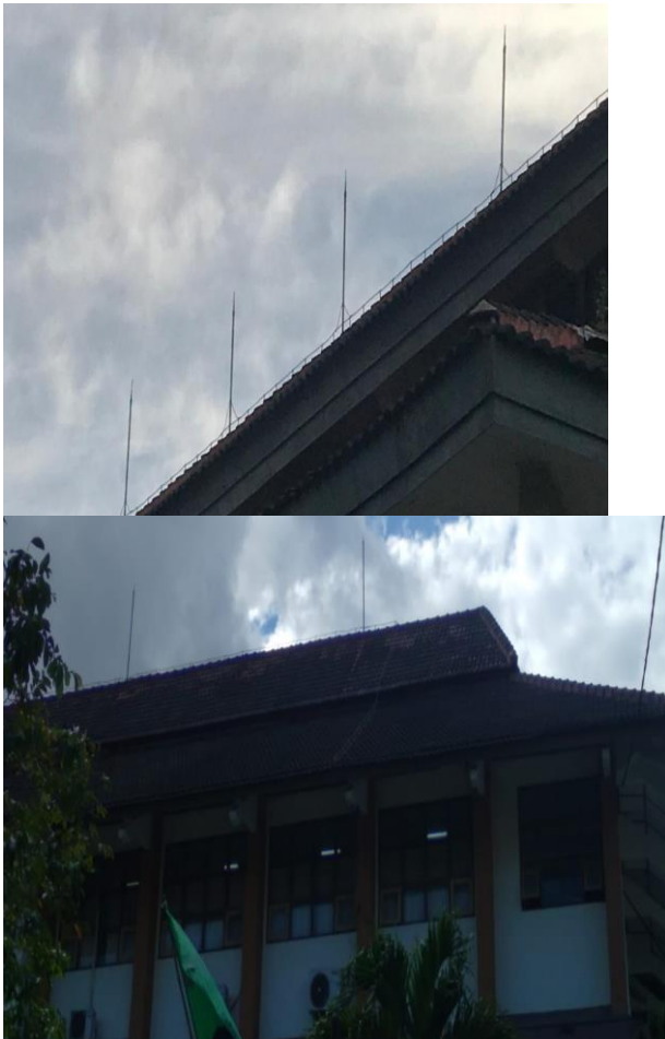
Figure 3. The Final Result of Installing a Lightning Rod
